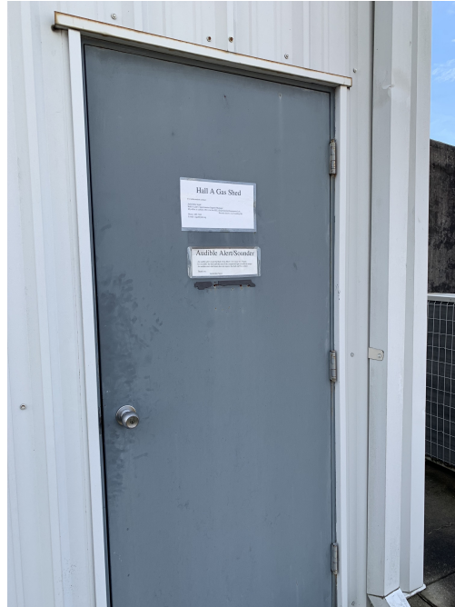
Figure 19: Hall A Gas Shed.
