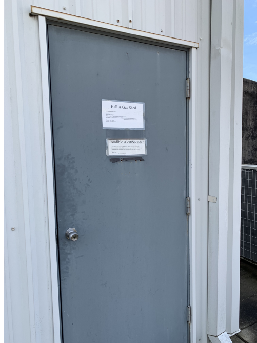
Figure 22: Hall A Gas Shed.
